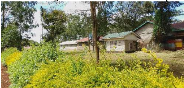
Plate 30: Existing transformer next to the workshops near the project site
